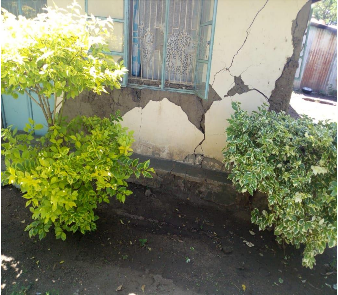
Plate 4. 1: Destruction of a house due to effects of flood in Magina (Source: Author May, 2019)
