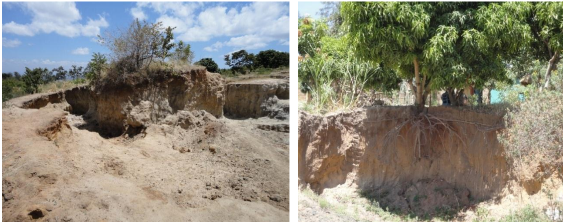
Figure 2. Impacts of sand harvesting on the farms at Manaja area.
