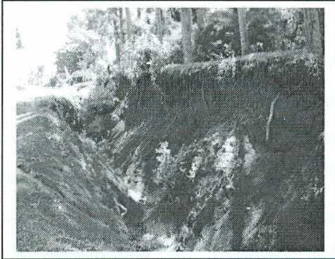
Plate 1: Gully erosion at the roadside Near Kiini dispensary
