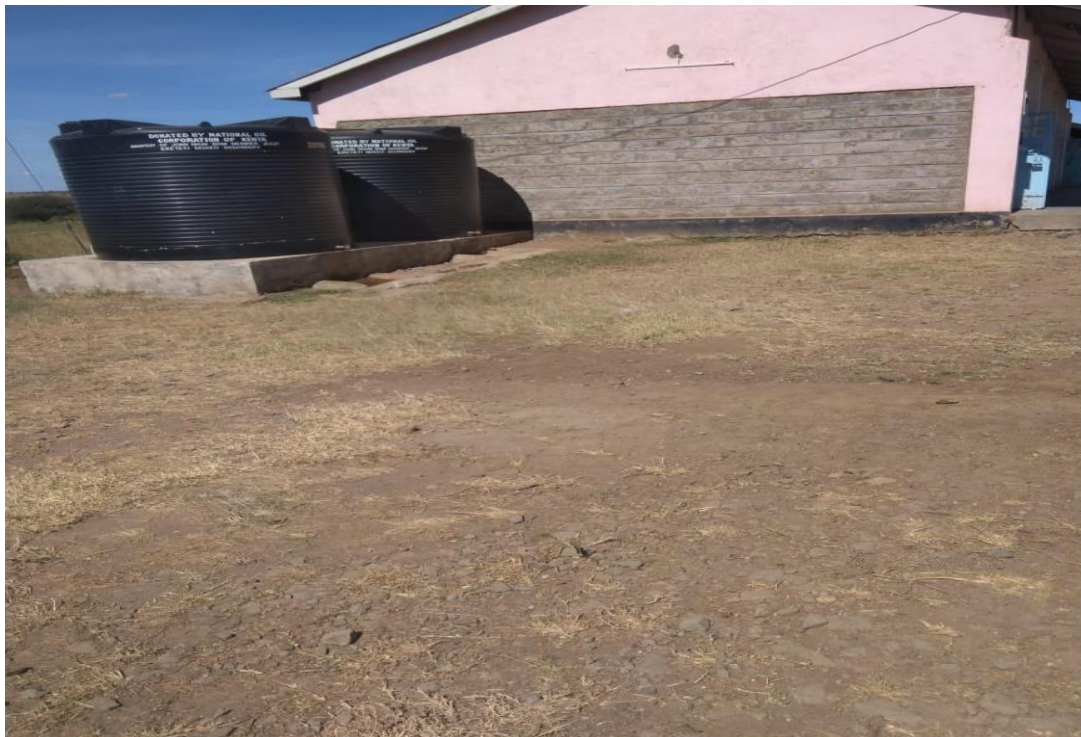
Figure 4.15: A Picture of Water Tanks (water harvesting)
