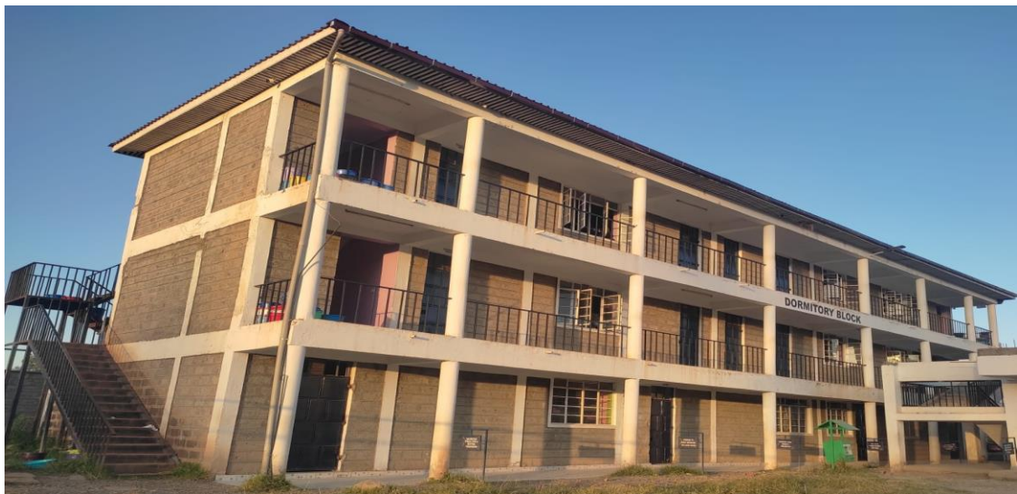
Figure 4.10: A Picture of a Dormitory Block
