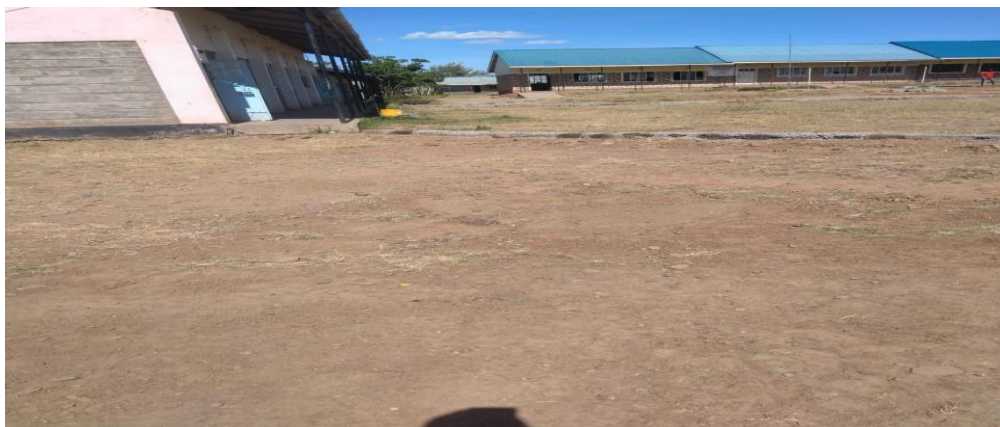
Figure 4.5: A well-maintained school premise in a Kajiado school
