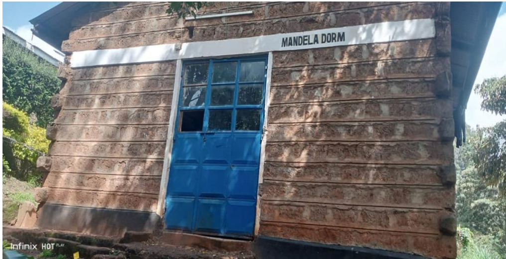
Figure 4.11: A Picture of a Dormitory Block
