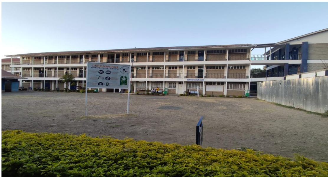
Figure 4.9: A Picture of an Administration Block and Classrooms
