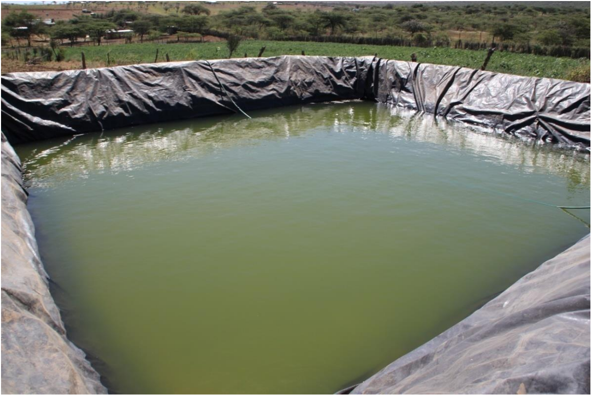
Plate 4.10: One of the polythene-lined dams that residents of Ngare Ndare settlement used to store water from Ngare Ndare forest. (Source: Researcher, 2016)
