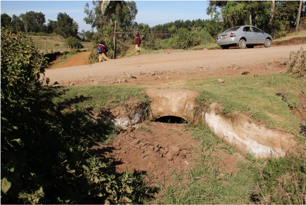
Plate 4.5: Karuai culvert in Kisima settlement of Ngare Ndare study site.
