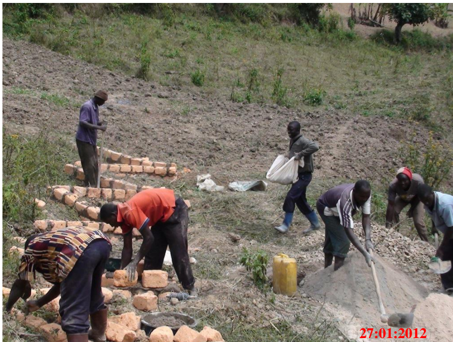
Plate 3.1: Constructing runoff plots
