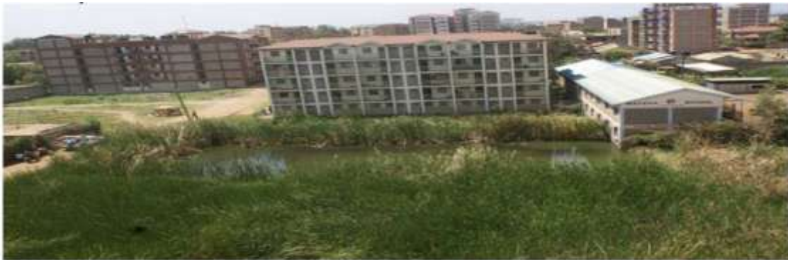
Houses constructed on an area with riparian vegetation in Juja, Kiambu County Source: NECC, 2018 (Photo taken in March, 2016).
