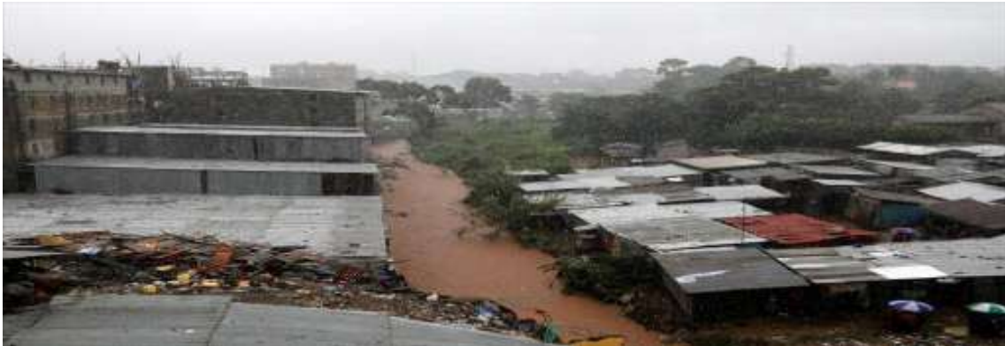
Figure 5.1: General view shows the Nairobi river flowing through the Huruma Estate neighborhood in Nairobi County, where a six-storey building had collapsed after days of heavy rain.
