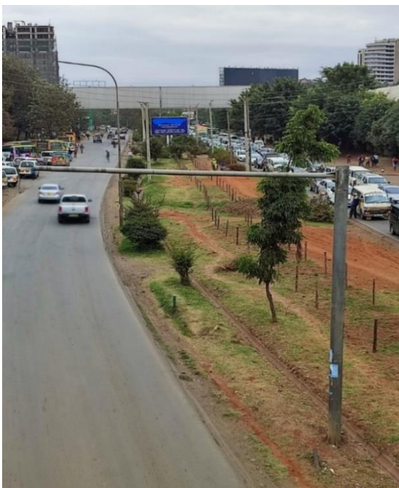
A CCTV site with cameras removed
