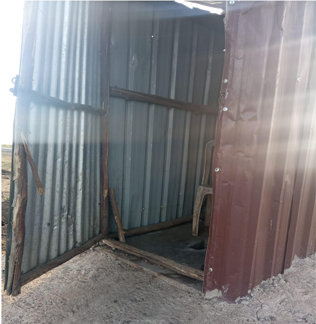
Plate 4.1: A temporal toilet structure in the area (Source: Author, 2022)
