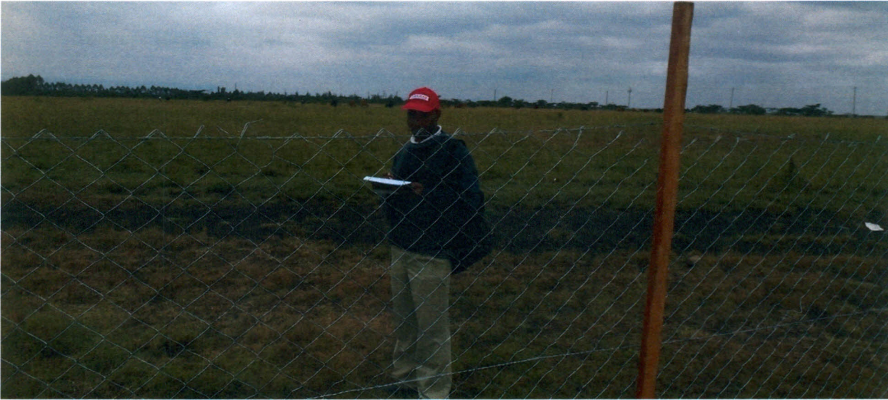
Plate 2: A newly constructed chain-link fence
