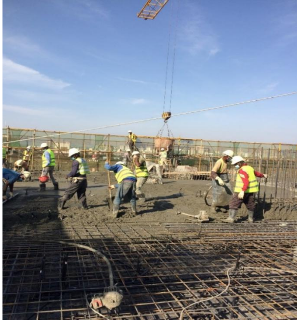
P.P.E.s compliant workers doing concrete works at the top most floor.
