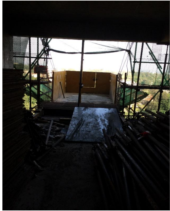
Material delivery area at the upper floor
