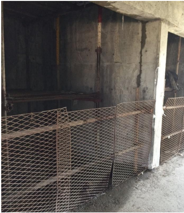
Lift shaft well barricaded
