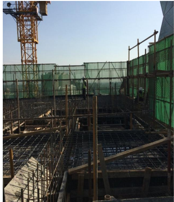
Well secured edges at the top most floor.
