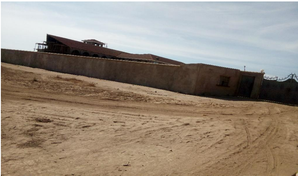
Figure 4.15 Ongoing construction work by a Sisters Congregation facility
