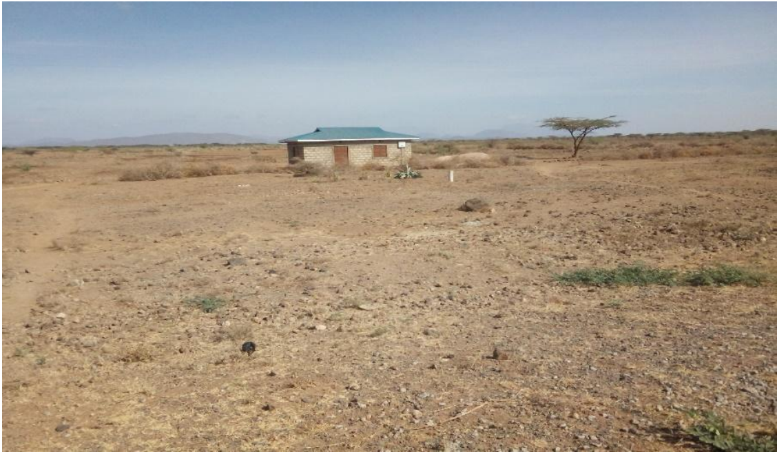
Figure 4.11: Construction of a permanent house to mark ownership
