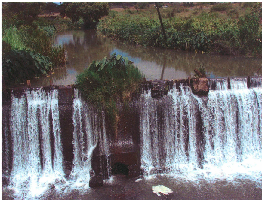
Plate5. 1: Water intake works on Ruiru River Source: Field data (2009)
