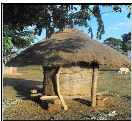
Figure 4.3 : Sisal-woven grass thatched granary for storing maize
