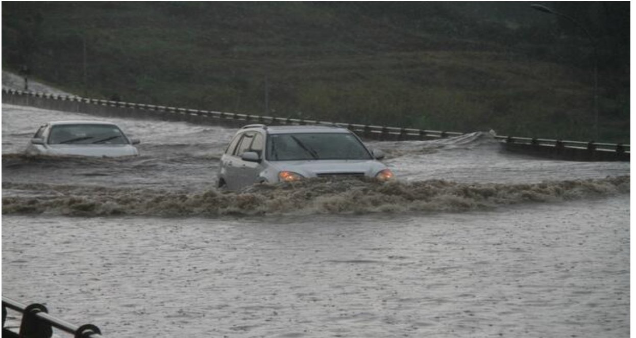
Plate 2: Drainage during rainy seasons
