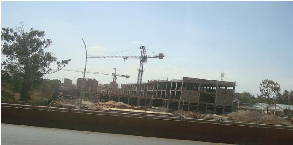
Plate 3: Construction of Thika Road Mall at Roysambu
