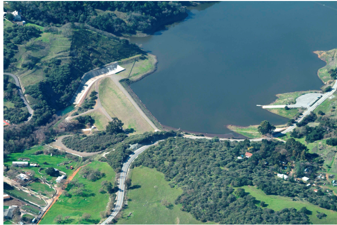
Figure 1.1: Chesbro dam and reservoir located in Llagas in Northern California . It can store 7945 acre-feet of water and has a surface area of 283 acres Source: www.valley.org/services/chesbrodam And Reservoir.aspx .
