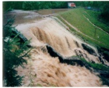
Figure 5.2: Glashutte Embankment dam overtopping on 12th August 2002 shortly before dam failure.
