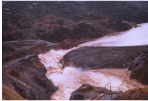
Figure 5.6: Failure of the 207 feet high Auburn Cofferdam on the American river on February 18 1986.
