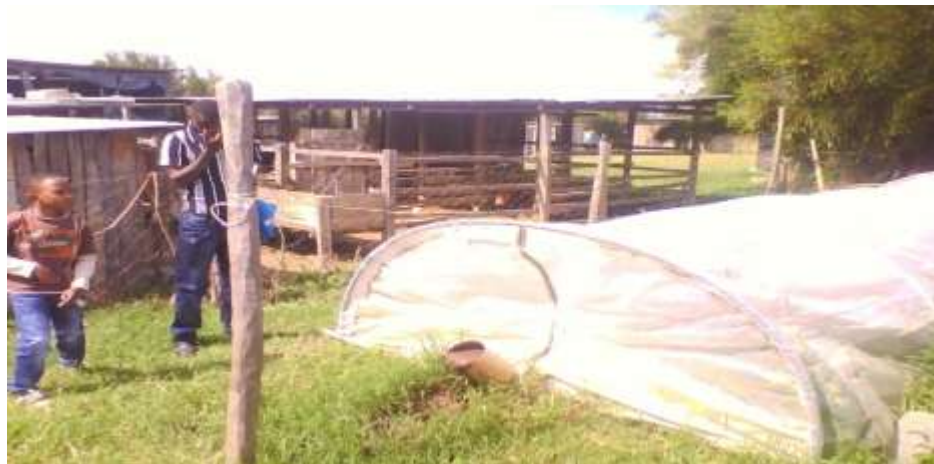
PLATE 15 a: An overflowing tubular bio-digester unit, spilling the slurry, overgrown with weeds, an expression of poor maintenance. Source: Field Survey (2015)
