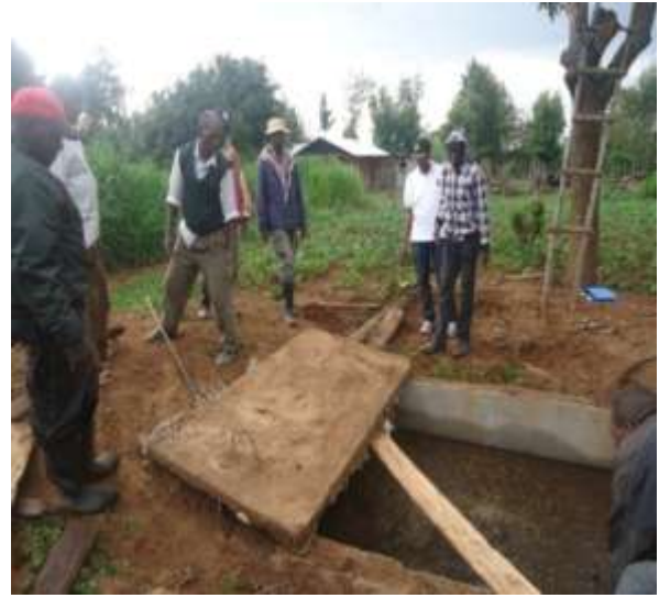
PLATE 11c Source: Field Survey (2015)
