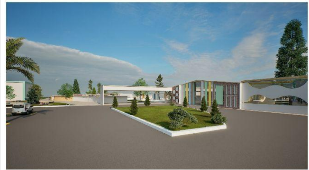
ENTRANCE THAT UNIQUELY SERVES BOTH JAMHURI ELEMENTARY AND KINDERGARTEN PEDESTRIAN WALKWAY ON THE RIGHT, VEHICULAR PARKING ON THE LEFT TOWARDS THE JAMHURI SPORTS COMPLEX THE FACADES ON THE ADMINISTRATION BLOCK IS MIRRORED
