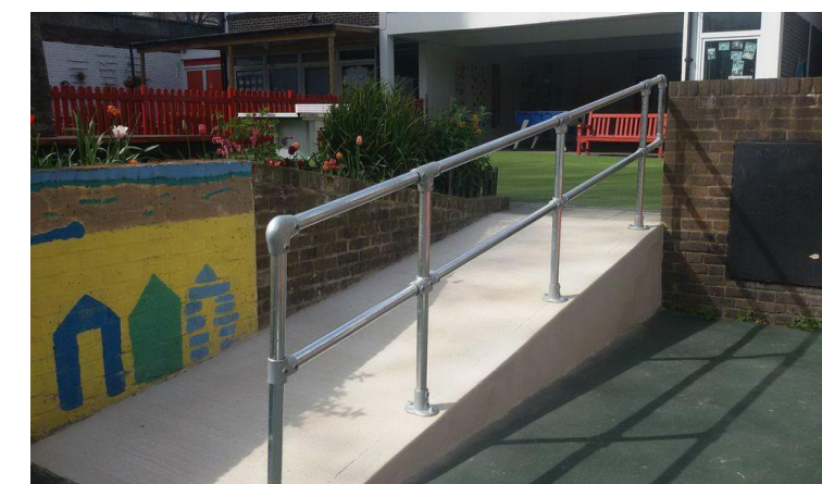
A Ramp to simplify access for users with different abilities.
