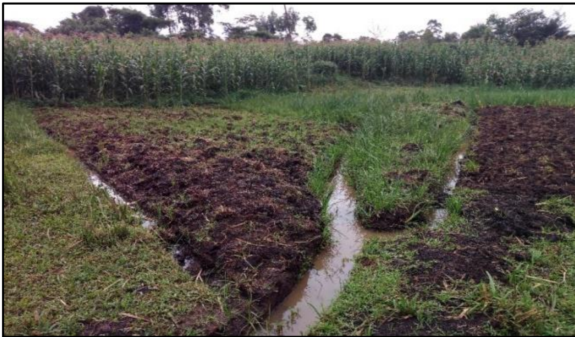
Plate: 4.3 Trenches Dug to divert Sinyerere river water into the nearby farms Source: Field Data
