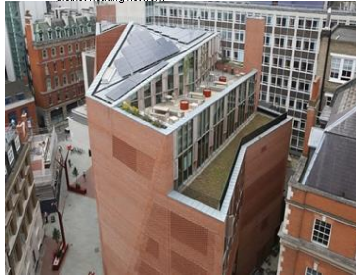
Source: Nigel Stead 2015 ;Photovoltaic system on the multifaceted roof
