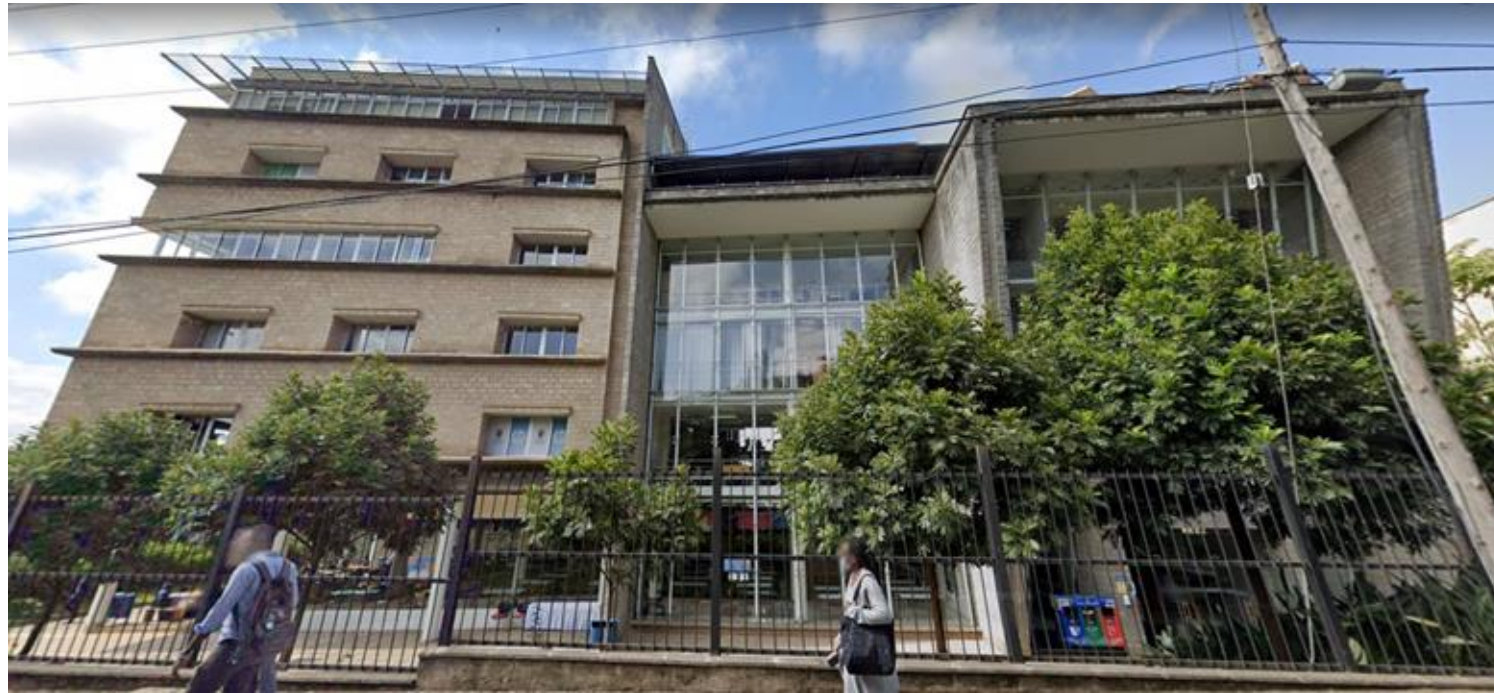
Image showing building façade Source:Ben Carson K.(2025)
