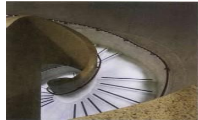
(Helical concrete stair. Source: Ros Diamond. photographer: Dennis Gilbert, 2015)
