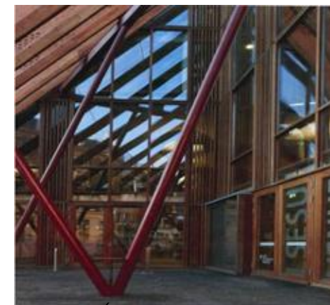
(a sealed glazed wall Source: Ros Diamond. photographer: Dennis Gilbert, 2015)
