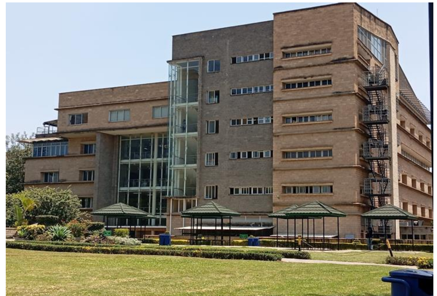
Image showing building façade Source:Ben Carson K.(2025)
