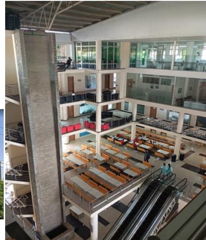
Image of evaporative wall Source: James K. (2025)
