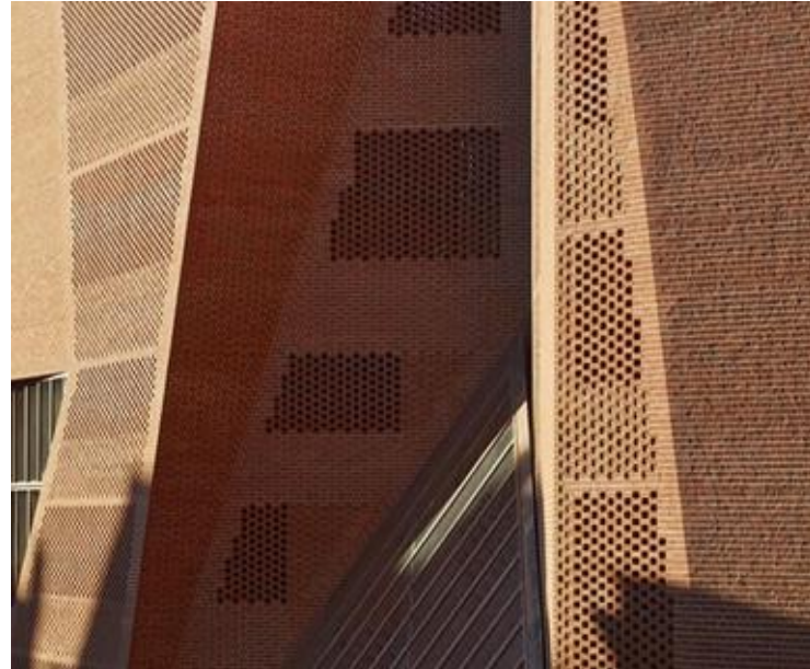
Source: Dennis Gilbert, 2015; Perforated brick facade
