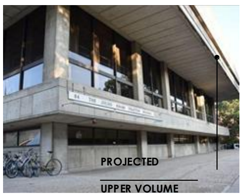
Figure Stratton student center. Source: https://culturenow.org/site/stratton-student-center/ The upper volume acts as an overhang, shading the building thus reducing solar heat gain.
