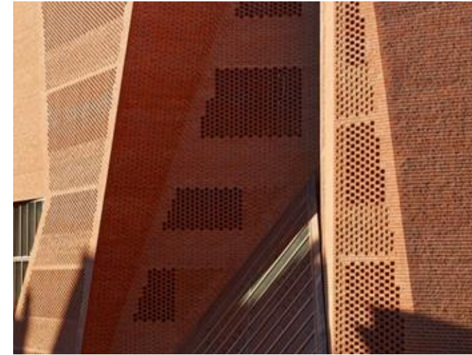
(source: Dennis Gilbert, 2015: perforated brick facade)
