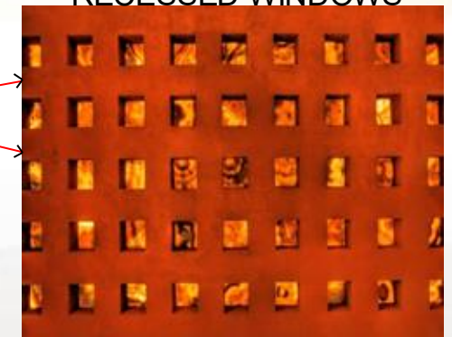
STUCCO WALLS WITH RECESSED WINDOWS
