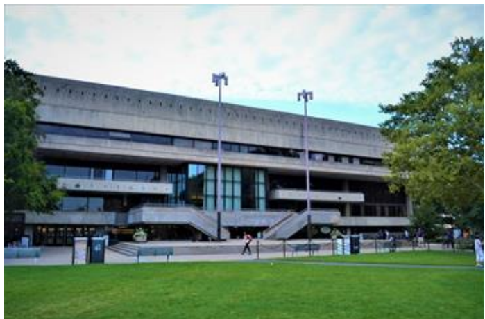
Figure Stratton student center. Source: https://sah-archipedia.org/buildings/MA-01-MT16
