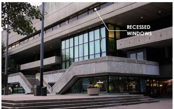
Figure Stratton student center. Source: https://culturenow.org/site/stratton-student-center/ The thin band of windows are recessed, reducing heat gain.
