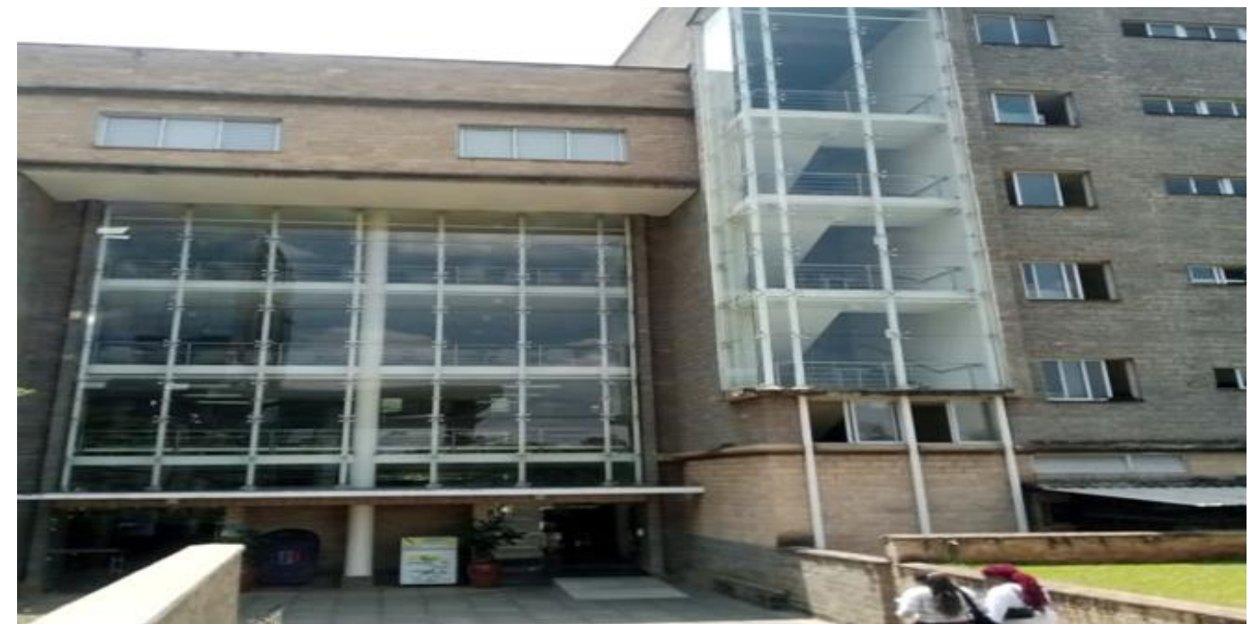
Image showing building façade Source:Ben Carson K.(2025)
