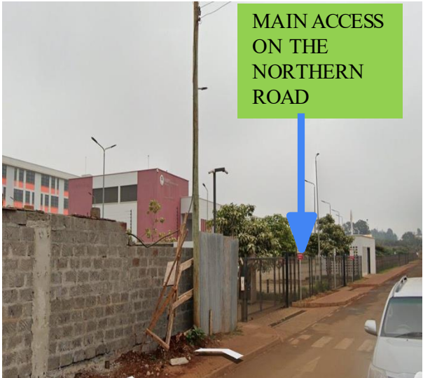
Maintenance at Sabis International school Runda Adapted from Weirimu, 2024. Rethinking The Future. https://www.re-thinking-the-future.com
