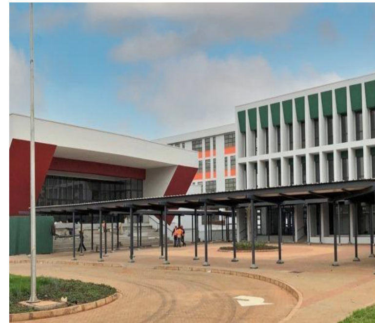
Image of the building blocks showcasing sun shading elements. : Waimu, R(2024). Rethinking TheFuture.
