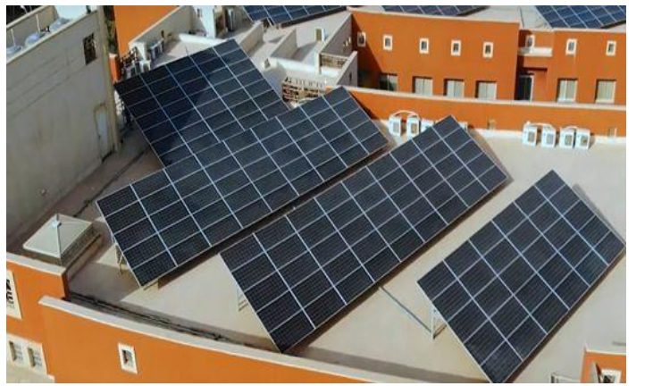
The images above and below show Solar panel layout on rooftop of Hayah International Academy Source: Presentation by Cairo Solar on how solar helped Hayah international academy save electricity. https://youtu.be/Wf24ZHvZGyQ?si=oMqP_gHws26AGjs0
