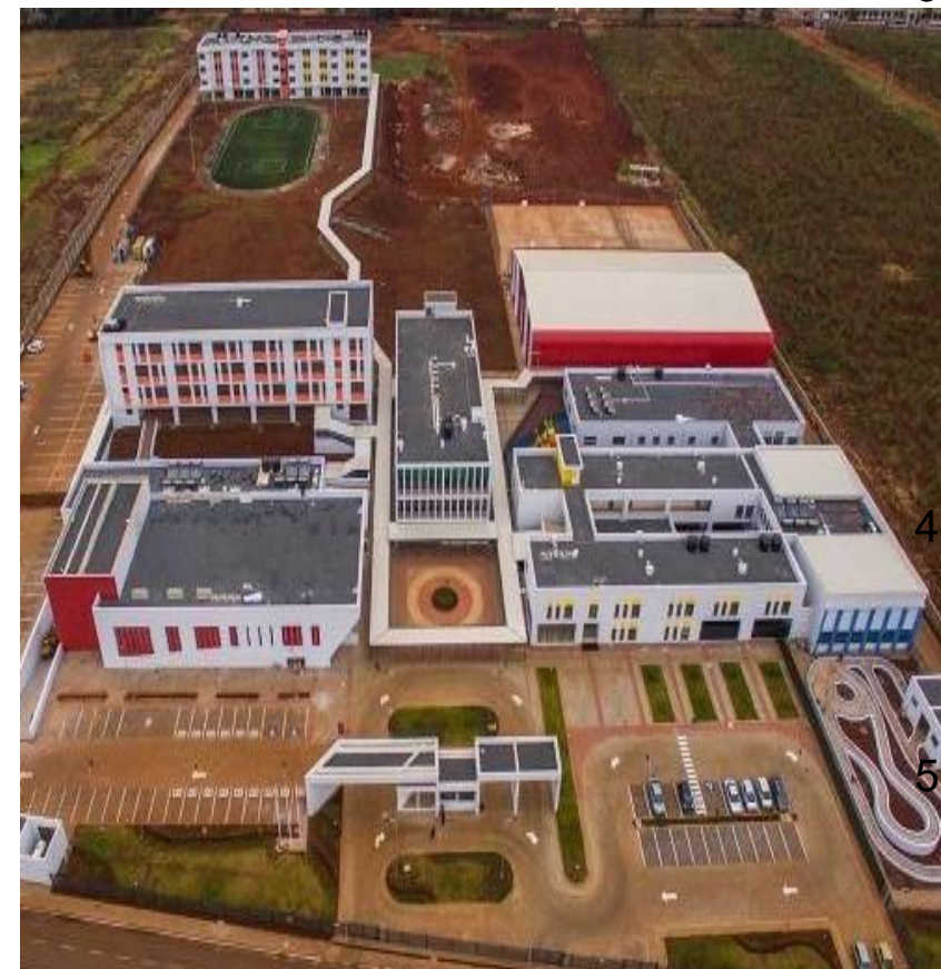
Image showing the site plan, showcasing the flat roof design and overall landscape of the school. Wairimu, R. (2024). Rethinking The Future .
