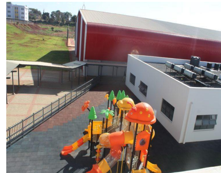
Overhead tanks to store recycled blackwater, Solid Green Consulting CC 2020. https://www.solidgreen.co.za/
