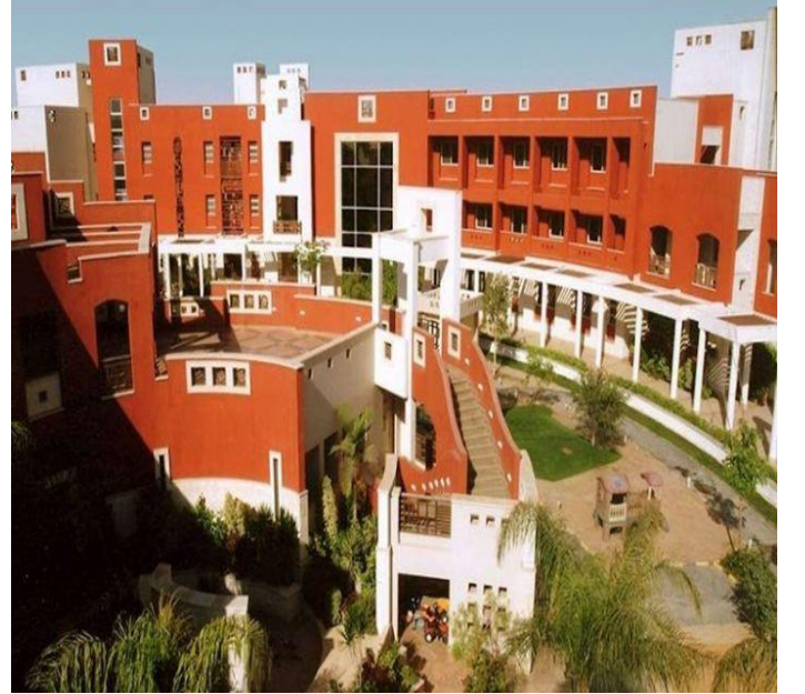
Fig 4: Kindergarten Source: Ramy Nassar, 2023
