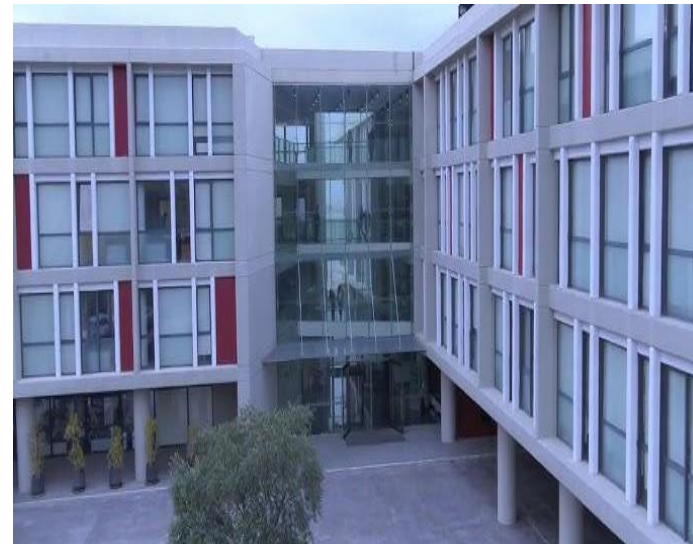
Classroom Façade. Adapted from sabisrunda.sabis.net 2024
