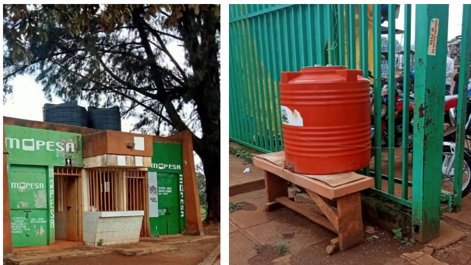
Plate 4.3: West market toilets and hand washing station
