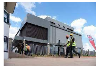
The Data Centre at Konza Source: Konza Technopolis, 2024
