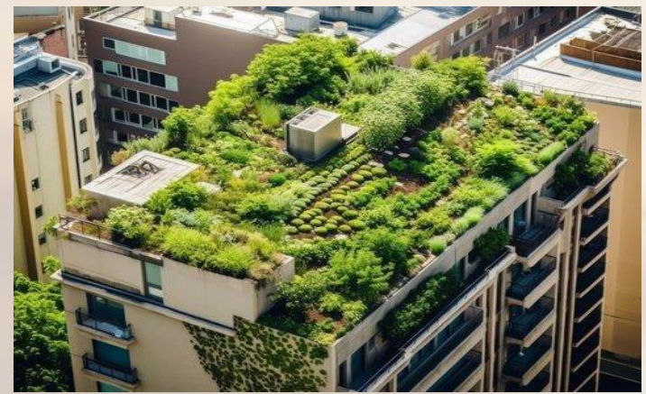
A rooftop garden. Source: Adobe stock..com( 2025)
