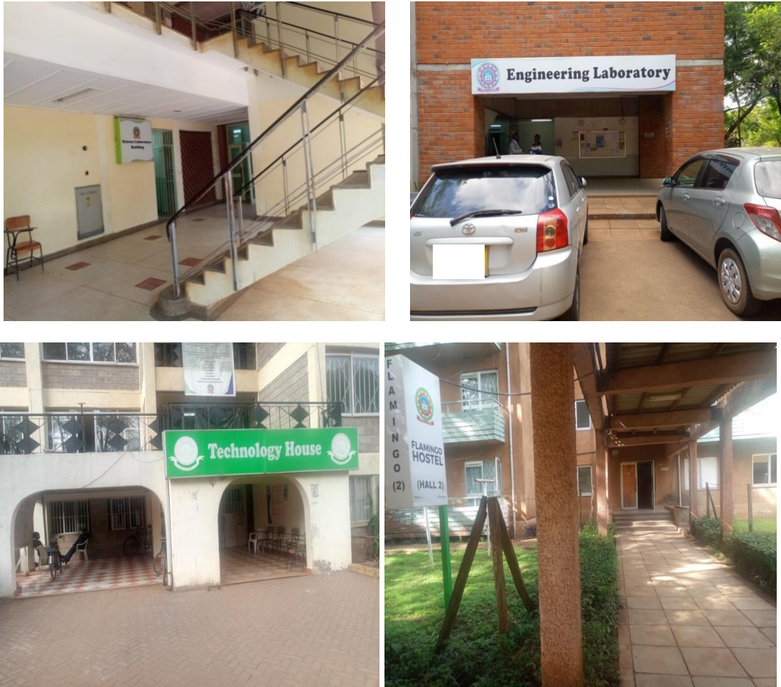
Figure 4.12 JKUAT Classroom and office Buildings with no adaptations for SWDs
