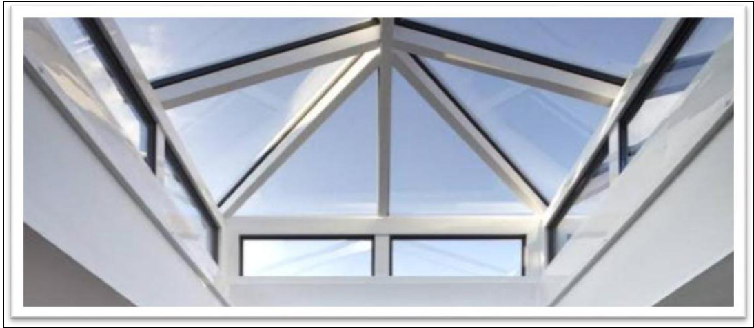
Plate 2.2: Skylight window and an Atrium
