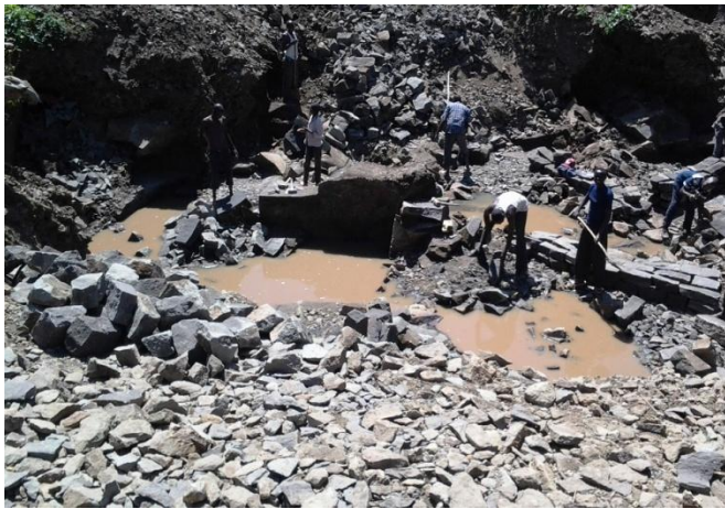
Mau/Kedowa, Kabao Quarry
