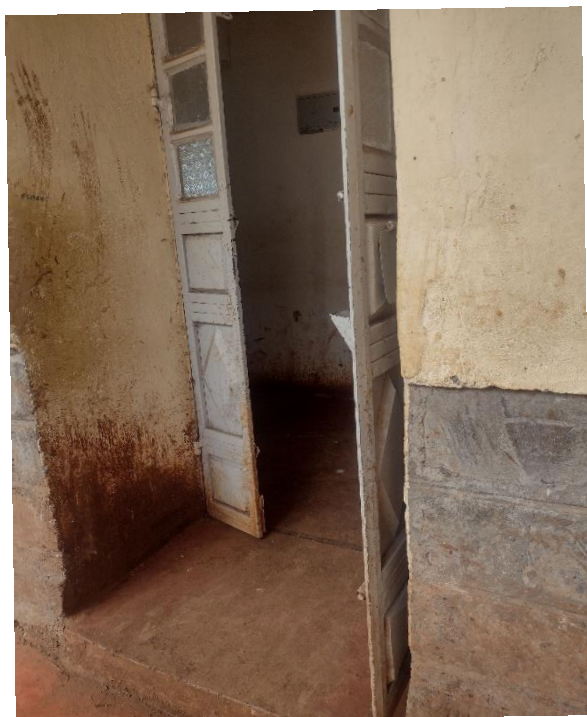
Figure 4.6: An example of a door opening towards outside and a spacious classroom
