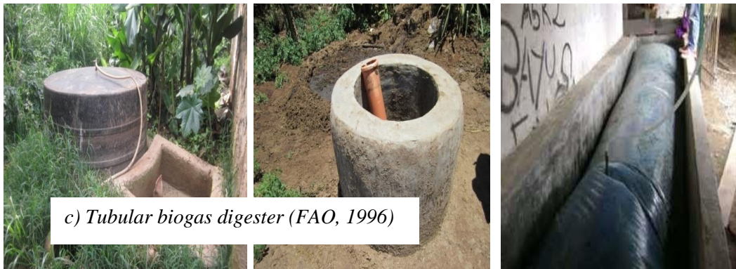
a) Floating drum biogas b) Fixed dome biogas digester c) Tubular biogas digester
