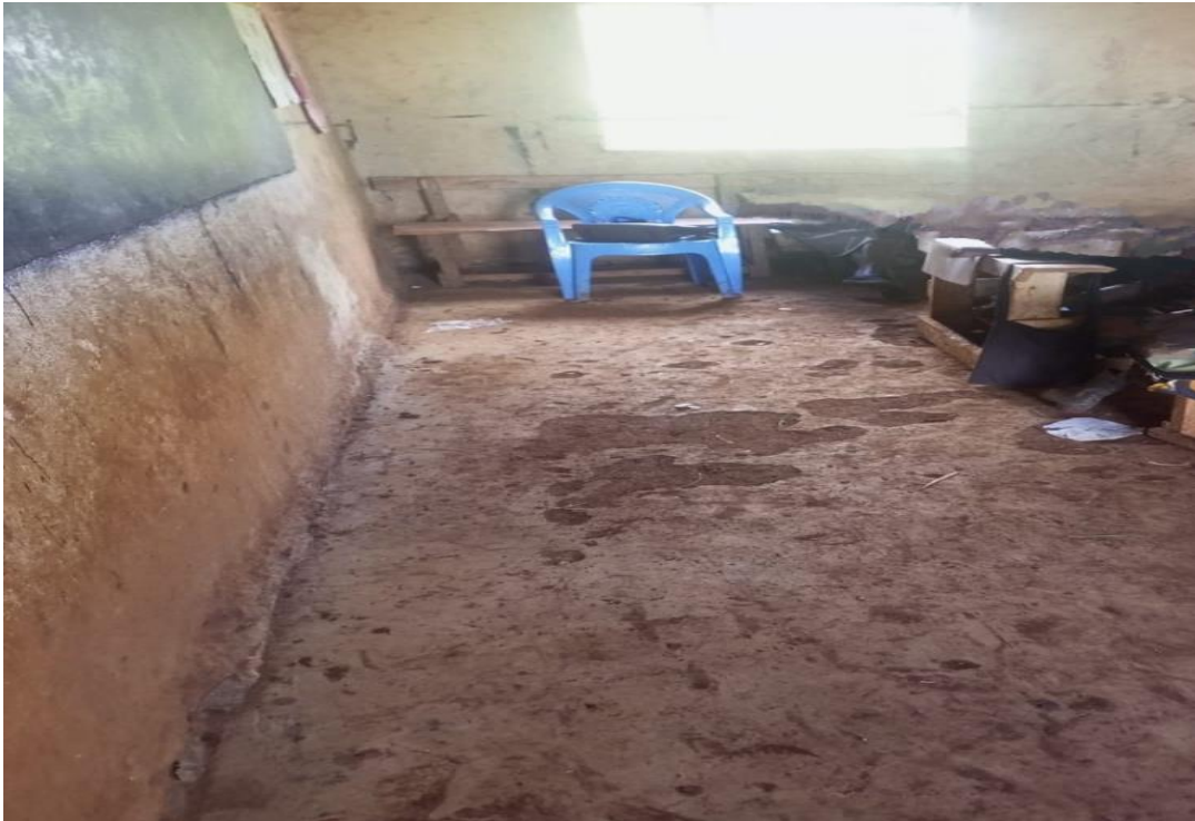
Figure 4.14: Condition of a classroom in one center
