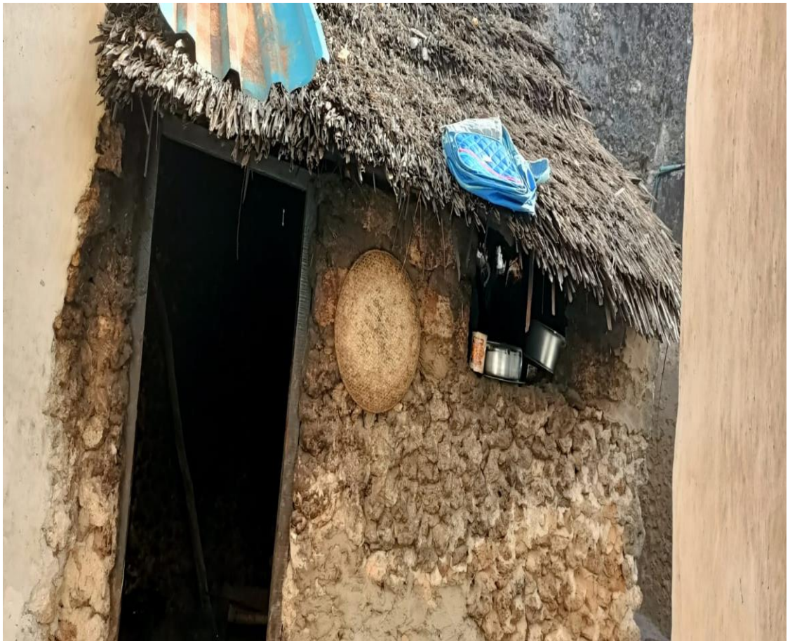
A Swahili house constructed using coral and traditional roofing in some parts (Picture by Author).
