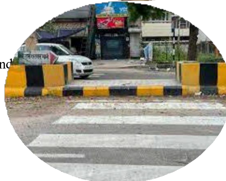
provision of zebra crossing and a pedestrian island on limuru road for safe crossing of students
