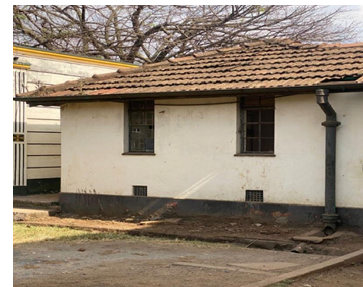
Image Showing the drainage channels from the roof
