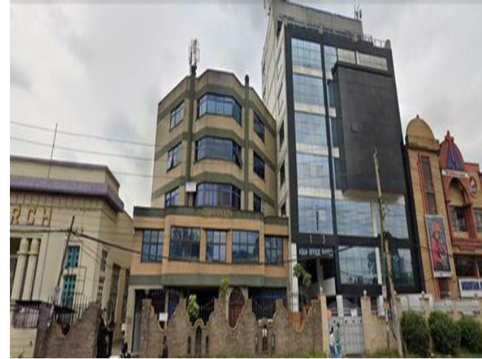
Aqua flats and offices Source: author, 2024
