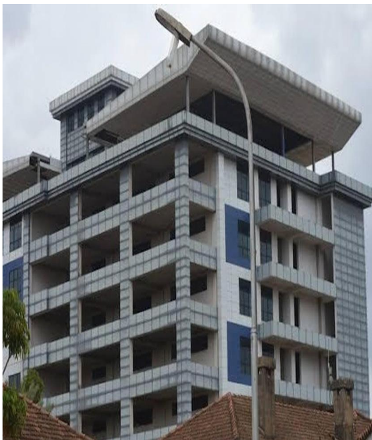
Image showing the KICD building
