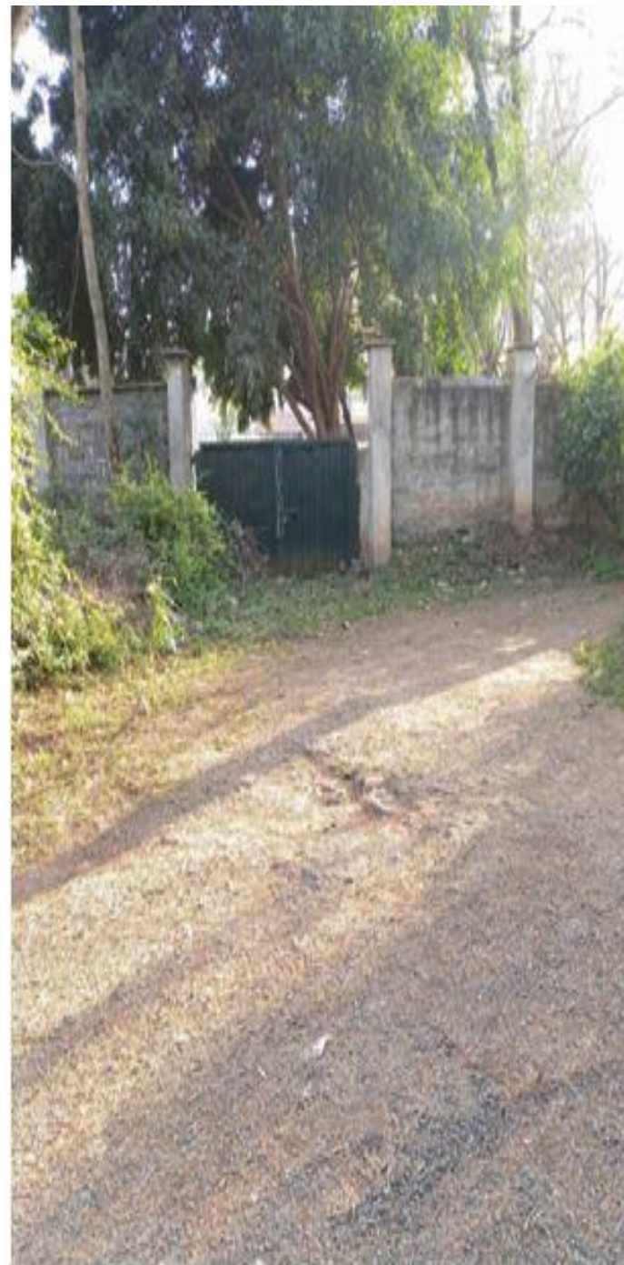
Abandoned gate Source: author, 2024
