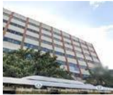
BUILDING WITH SLIDING WINDOWS
