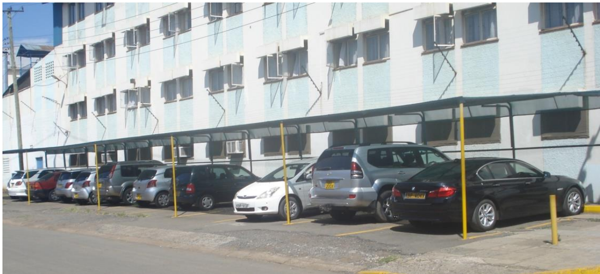
Plate 5-8: Parking with an improved shade to avoid corrosion of vehicle surfaces
