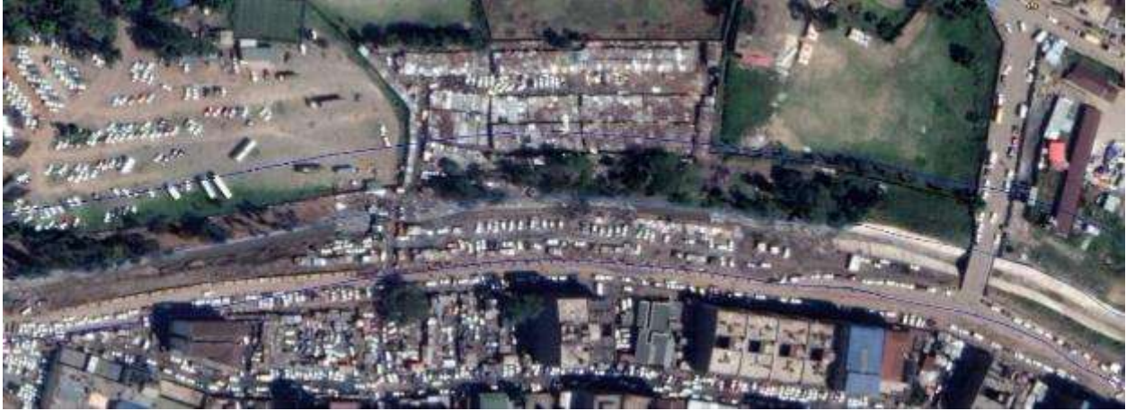
Figure 14. A section of Nairobi River at Grogan stretch characterized by garages at the riparian zone
