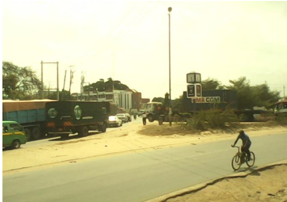
Plate 5.8: Showing a cyclist along the Kibarani hot spot but there is no even the cyclist path, hence he can lose control and get into the vehicles lane.
