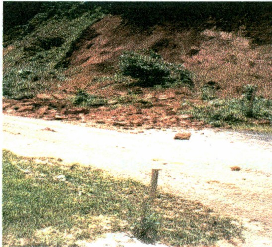
Plate 3.3: Landslides in Nyungwe Forest
