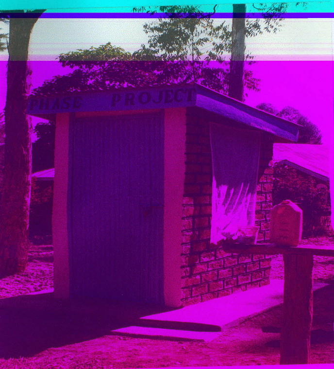
c) A school latrine (VIP) in good condition and a leaky- tin on the side
