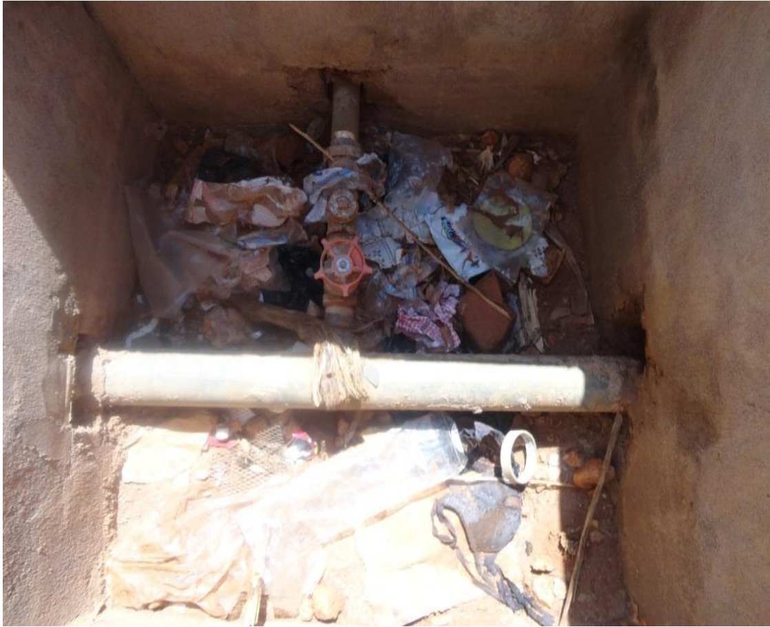
Plate 9: T-Point along Kamuwongo-Tyaa Kamuthale pipeline
