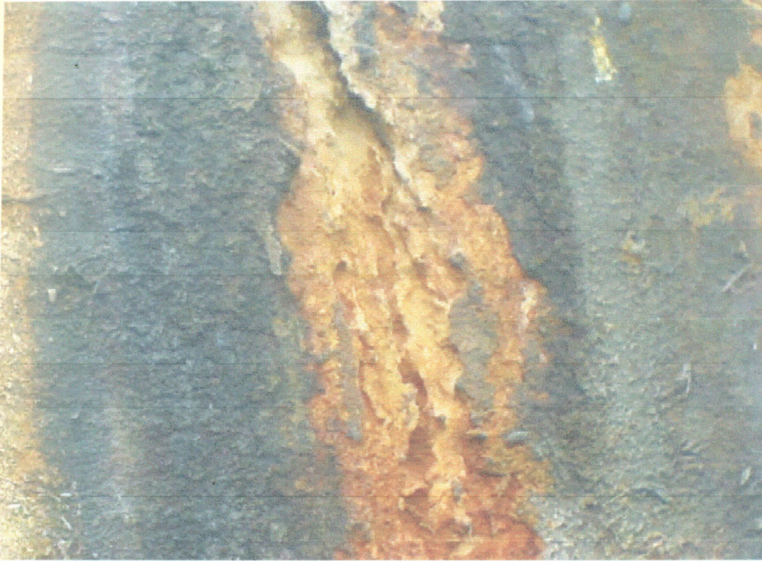
Plate 2.1: Concrete Cracking due to Rebar Corrosion Products. Picture of a Grilled Concrete Wall of the Simon Building Corridor of the University of Manchester
