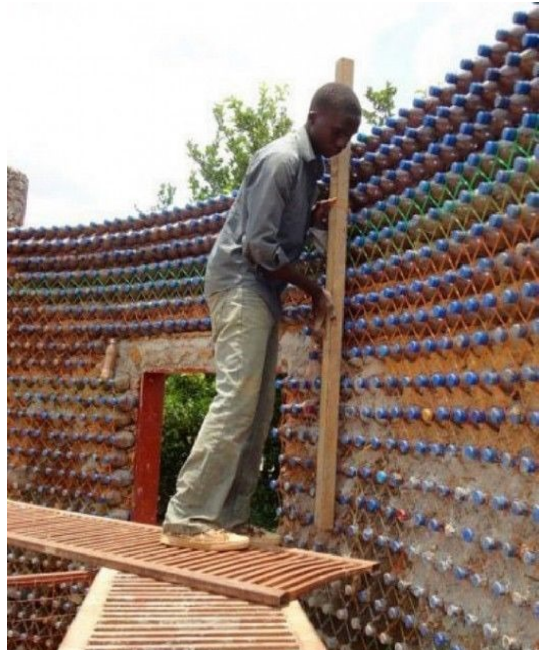
Figure 79 Construction with plastic bottles in Nigeria, Source BBC 2008
