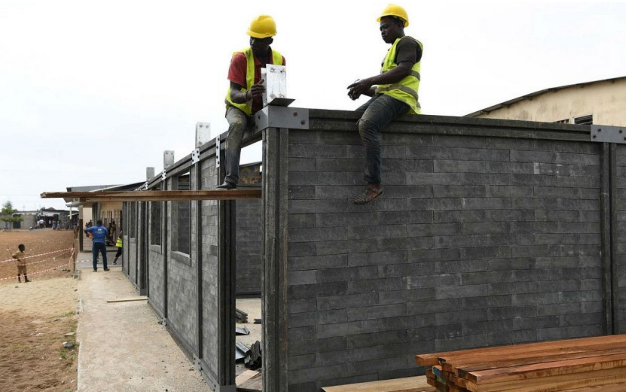
Figure 1 Construction using plastic blocks by Timao Group. Source Author 2023.
