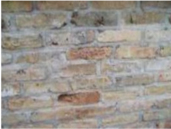
Figure 63 Brittleness characteristic of the brick
