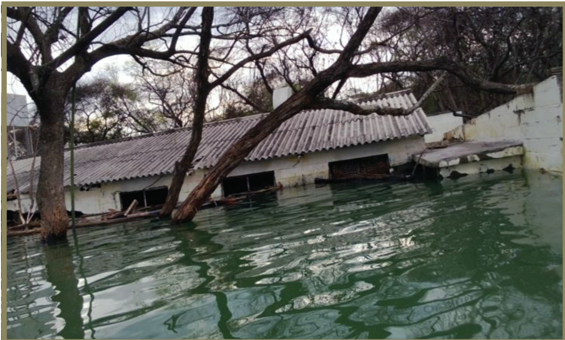
Submerged Lake Baringo Club Lodge facilities.
