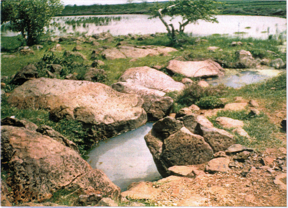
Plate 7: A rock catchment dam. On the background is the rock catchment dam while on the foreground is a seasonal spring. These dams are built near seasonal springs for replenishment.
