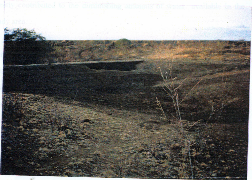
Plate 8: A check dam with concrete weir in the dry season. The dam is heavily silted (as can be seen on the middle ground) and will soon be rendered useless if not dredged.
