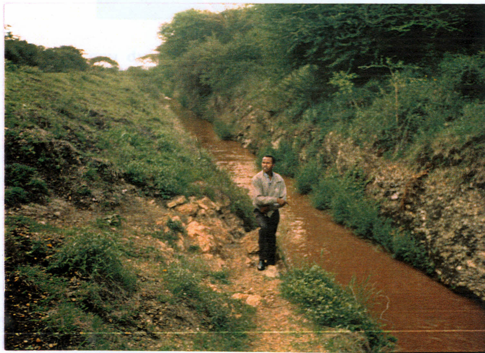
10: A well protected section of the Yatta canal.
