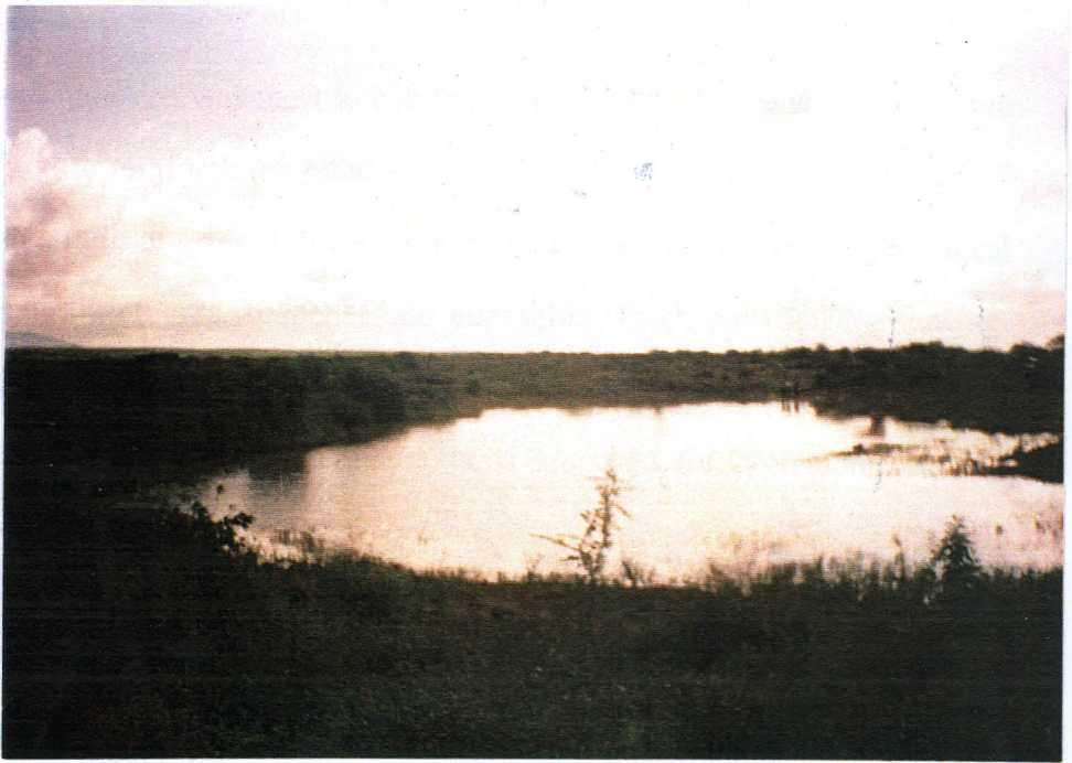
6 (a): A well protected E earth dam in the rainy season with vegetation around it.
