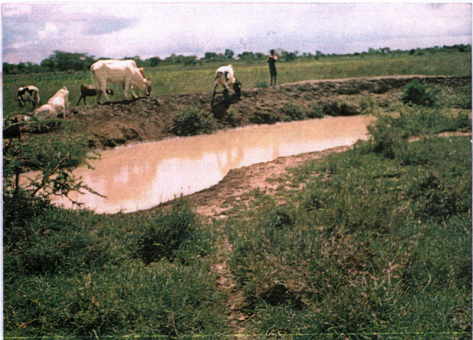
Plate 5 (b): The same earth dam (5a). The drinking point is eroded by animals.
