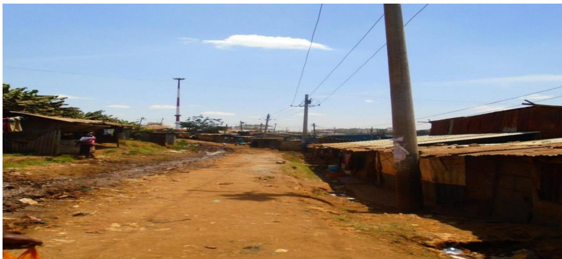
Figure 4.12: Electricity connection in the slum
