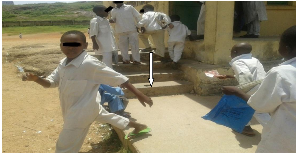
Picture 4.3: A Classroom with Steps instead of Ramps
