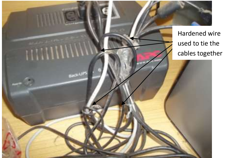
Plate 4.2: Hardened wire used to tie cables together in one of the libraries.
