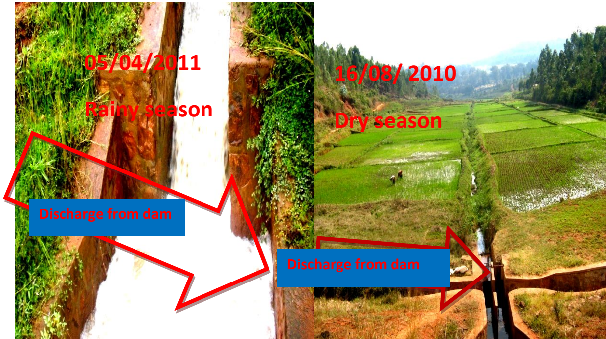
Plate 4.4: Rusurirwamujiya outlet dam (the main canal upstream) in the rainy and dry seasons
