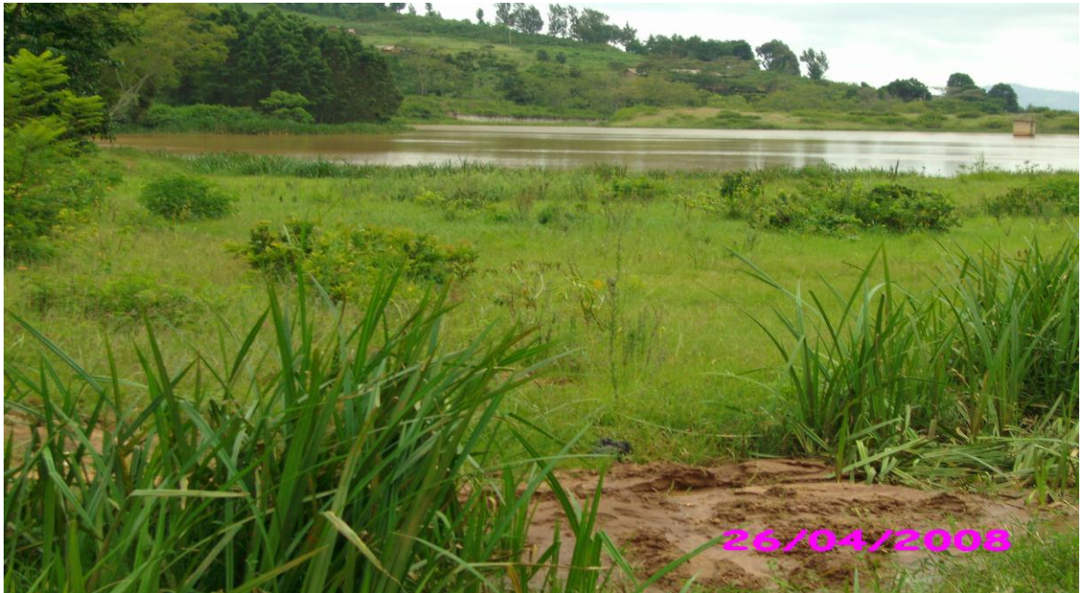
Plate 4.1: Rill erosion in Muooni dam site
