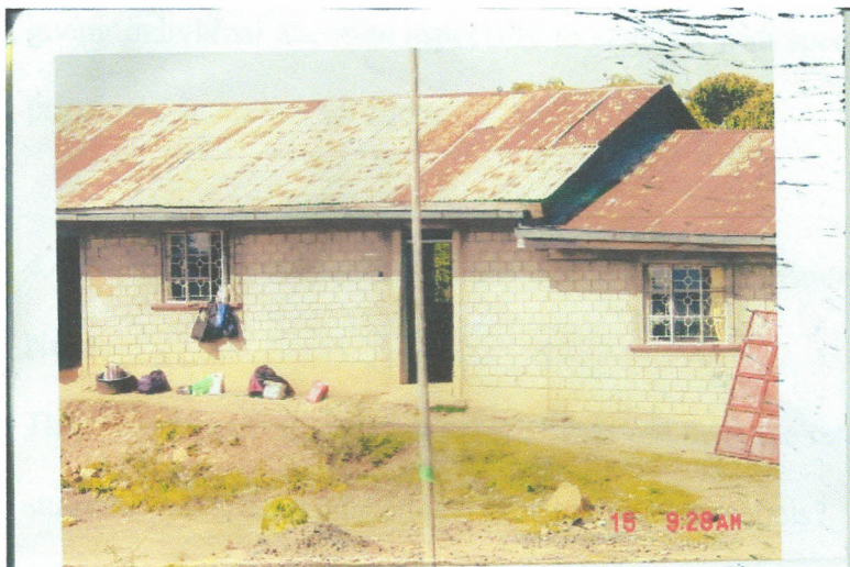
Figure 4.2: The condition of doors as entrance to classrooms
