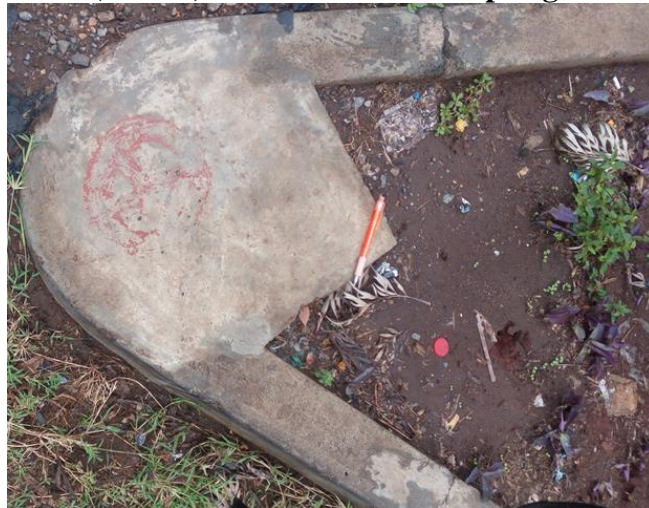
Top edge of slab (GCP 7)
