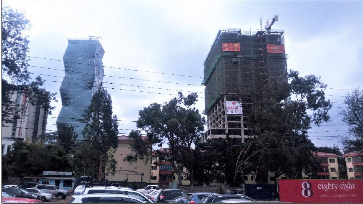
c) Construction of high rise buildings along Fourth Ngong Avenue
