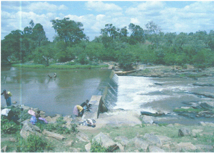
Plate 4.2: A Weir for Chebaraa Irrigation Water Intake at Kaboson Photo taken, 17 th December 2014
