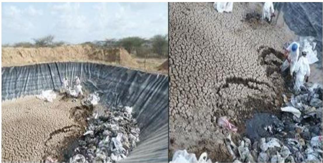
Plate 4.10: Drill cuttings temporary storage in a reserve pits in Twiga 1 (Source: Tullow BV Kenya Ltd., 2017)
