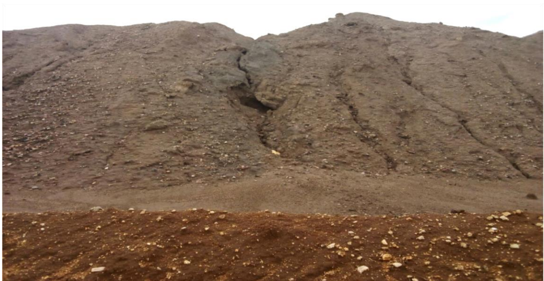
Plate 4.15: Tunnels of eroded mud cuttings by the surface runoff (Photo: Researcher, 2017)
