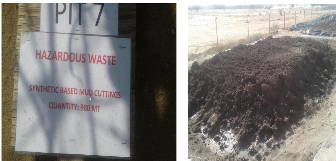
Plate 4.12: Reserve pit 7 full of drill cuttings in Twiga 1 (Photo: Researcher, 2017)
